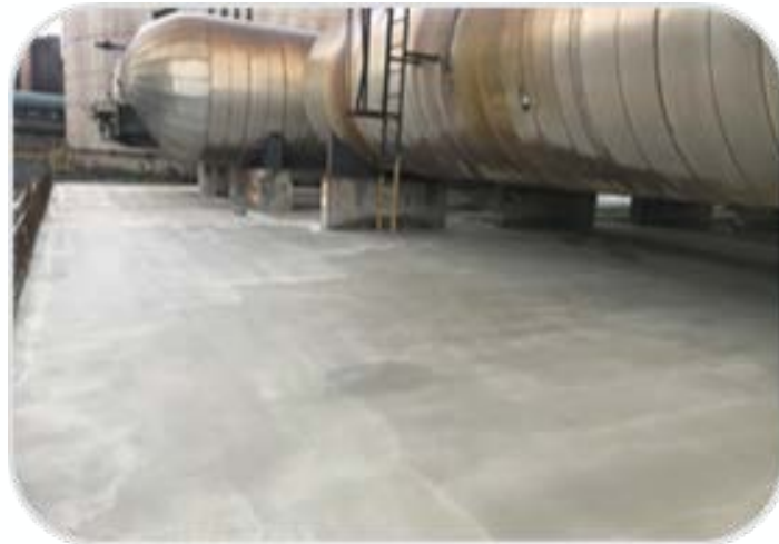
New Secondary Containment on Waste Oil Storage Tanks
