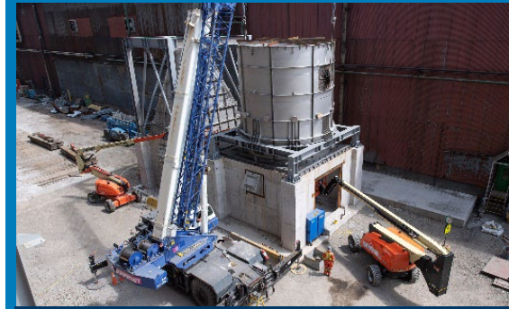
Quench tower assembly is underway
