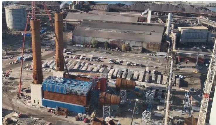
Stacks on Fume Treatment Plants installation
